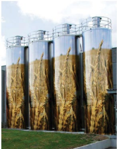
Welded Outdoor Silos
