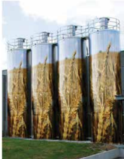
Welded Outdoor Silos
