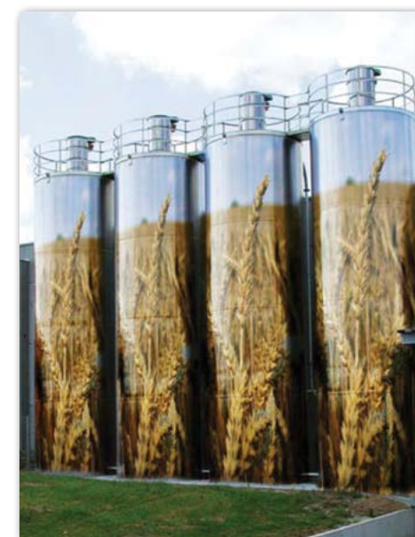
Welded outdoor silos
