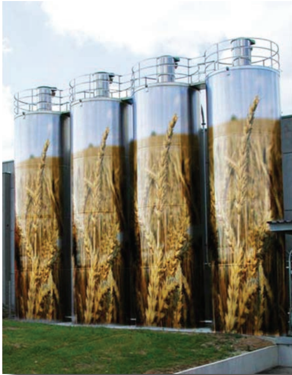
Welded outdoor silos
