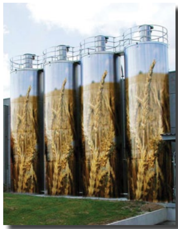
Welded outdoor silos
